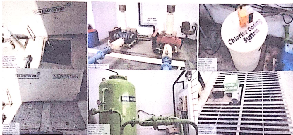
Sewage treatment Plant
